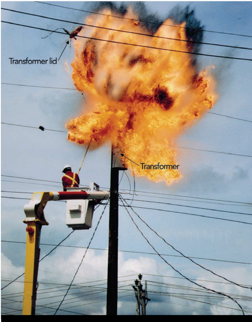
This is the possible result of reclosing on a transformer with an internal fault. This photo was staged at a utility test lab with a mannequin, not a line worker, and the reclose onto the line voltage was done remotely.
